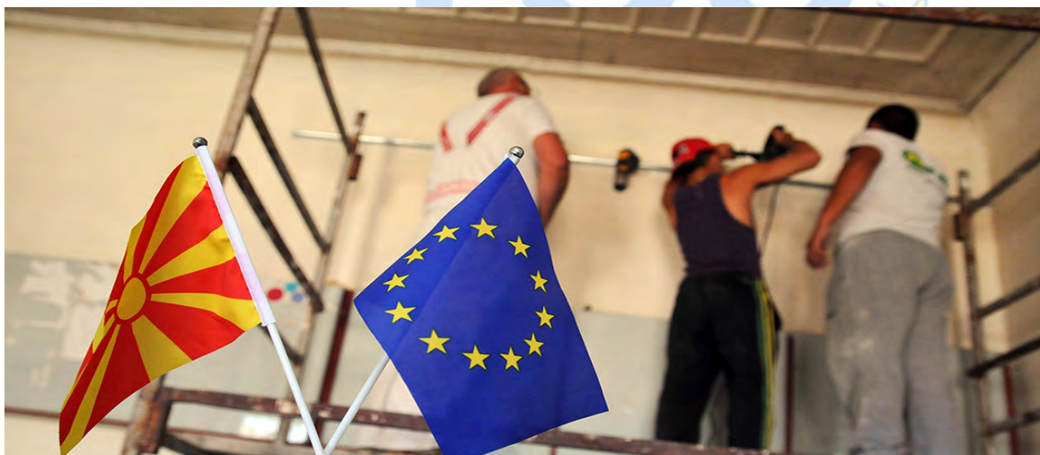
Roma men gaining practical skills in drywall construction in Prilep.
